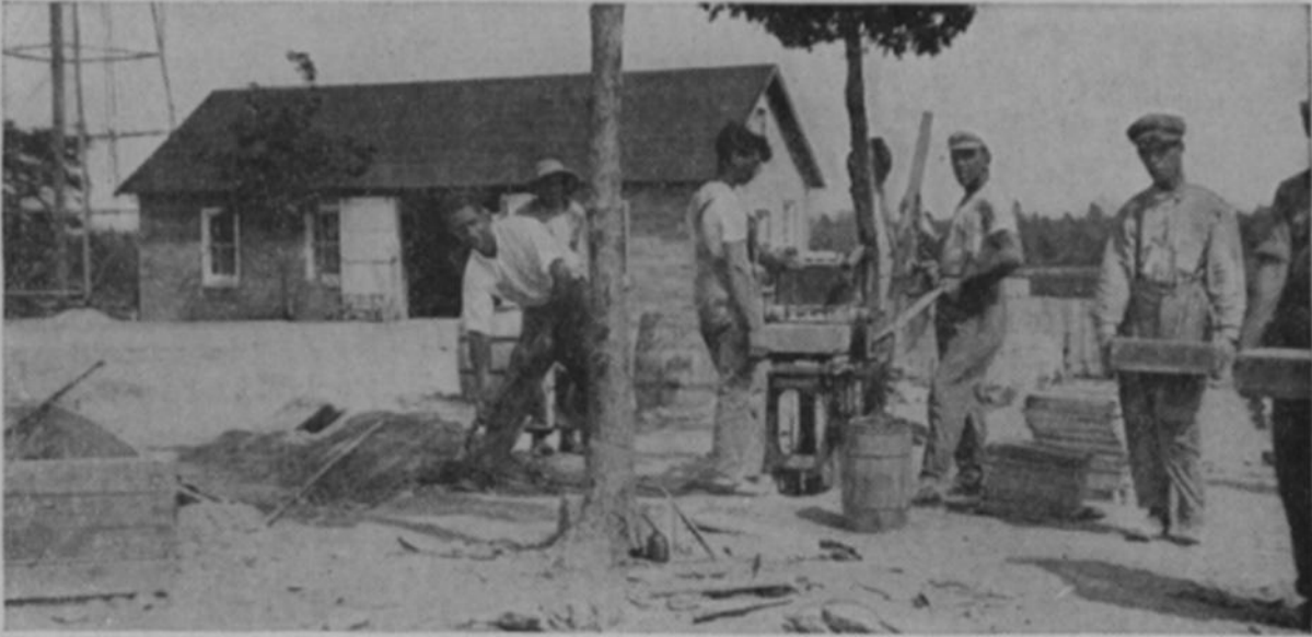
MAKING CEMENT BLOCKS
